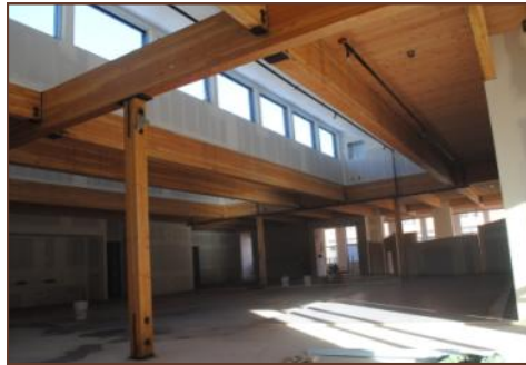
A sneak peek inside the New Castle remodel in mid December reveals natural light and beautiful beams.
